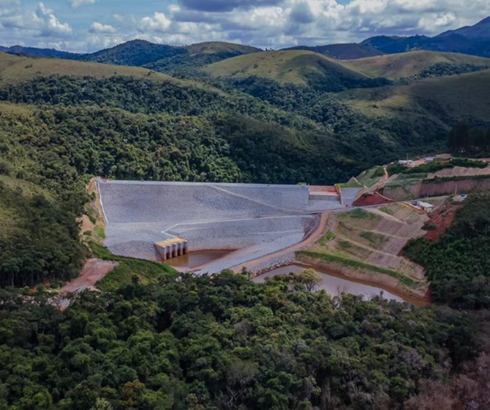
B3/B4 back-up dam, delivered in 4Q20
